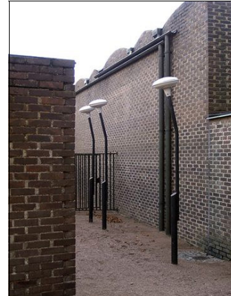
The bent lampposts around the exterior of the chapel are a signature feature of Lewerentz's work.
